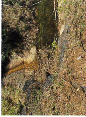
IMG_403-View Upstream Flow Present
