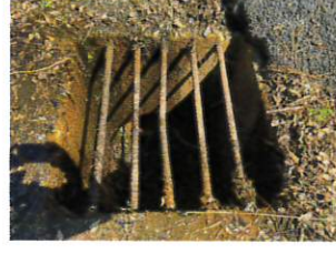
IMG_0412-View Upstream Debris Removed
