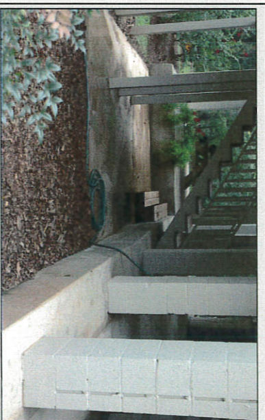
A new 3-foot concrete slab foundation was poured before elevating this house on cinder block piers to mitigate against flooding.
