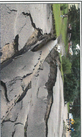
Drainage systems obstructed with trash or other debris can cause an increased risk of flooding since the floodwaters have no place to drain. The increased flooding caused by those obstructed drains can severely undermine the local roadway infrastructure structure, leading to potential health and safety hazards.
