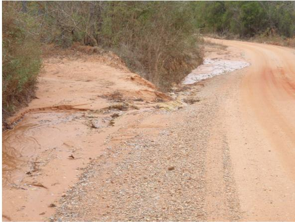
Photo 3: Example of failed “turn-out”.
