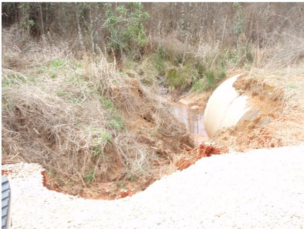
Photo 5: Lack of adequate outlet protection.
