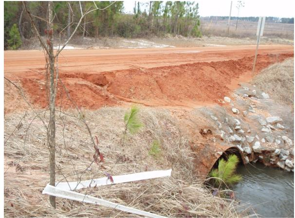
Photo 4: Example of fill placement without BMPs.
