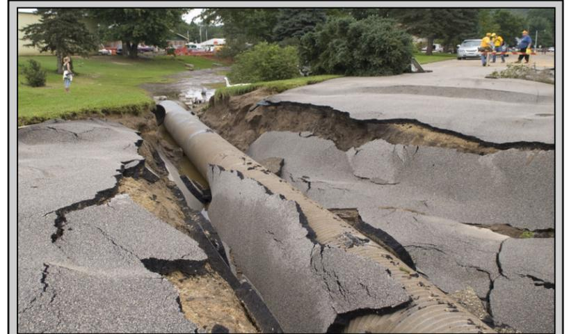
Drainage systems obstructed with trash or other debris can cause an increased risk of flooding since the floodwaters have no place to drain. The increased flooding caused by those obstructed drains can severely undermine the local roadway infrastructure structure, leading to potential health and safety hazards.
