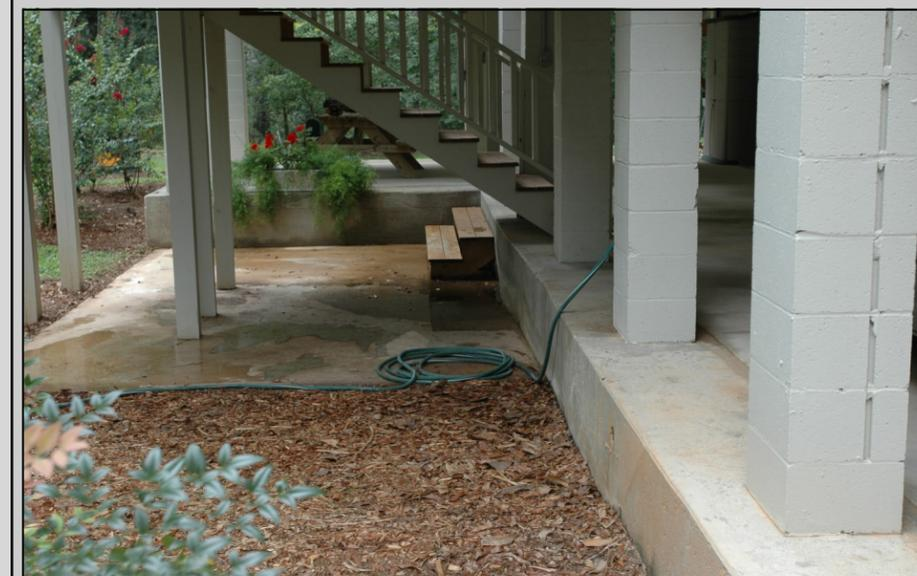
A new 3-foot concrete slab foundation was poured before elevating this house on cinder block piers to mitigate against flooding.
