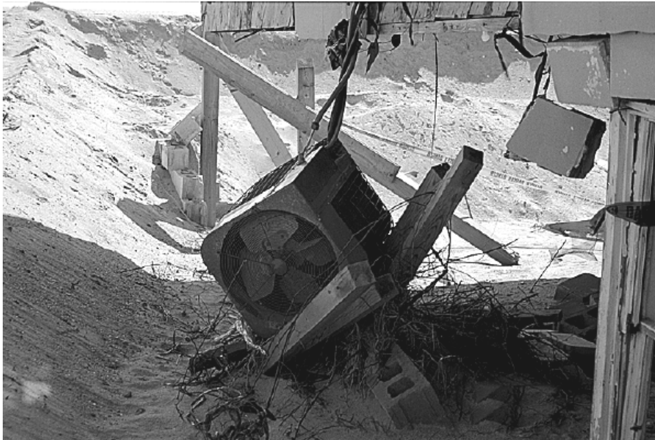
Figure 3.1.3A: Electric heat pumps dislodged from their stands by velocity flow during Hurricane Fran in Topsail Beach, North Carolina, in November 1996
