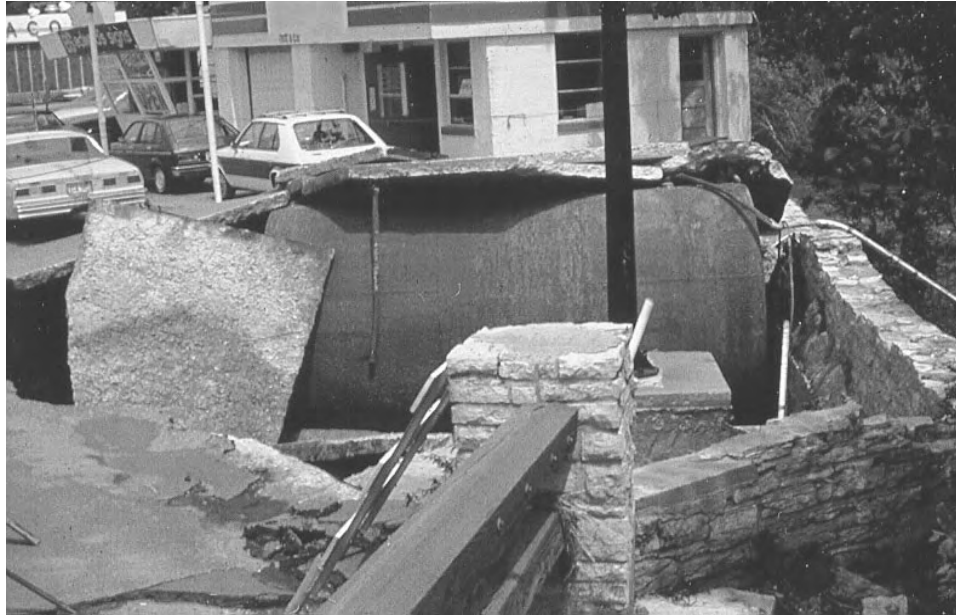
Figure 3.2.3.1A: Tank lifted by buoyancy forces
